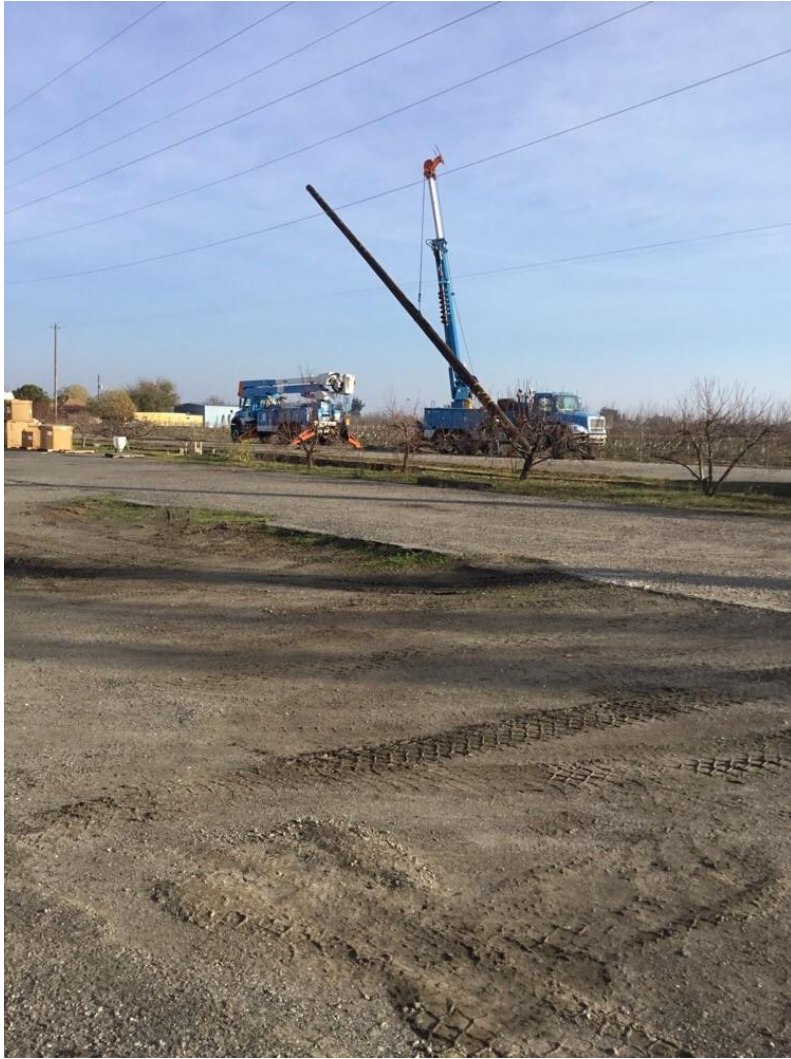
Photo 2: Crews removing a snub pole at structure 4/39.
